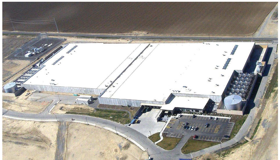
Microsoft Datacenter in Quincy, Washington
